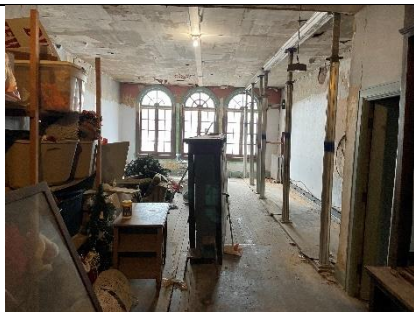
Second Floor – Temporary Shoring
