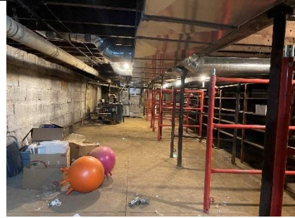
Basement – Temporary Shoring
