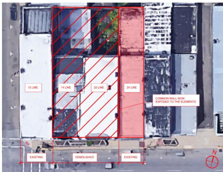
Figure 1: Aerial View (Pre-Demolition of 14 LWE and 20 LWE). Image is from Google Earth.
