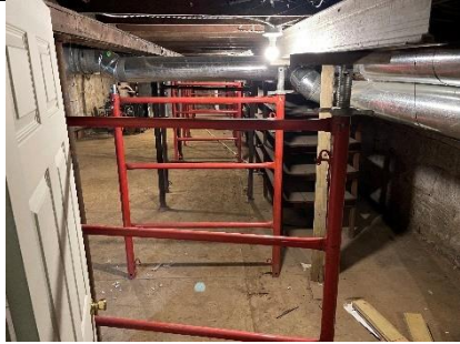
Basement – Temporary Shoring
