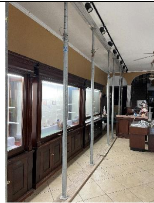
First Floor – Temporary Shoring
