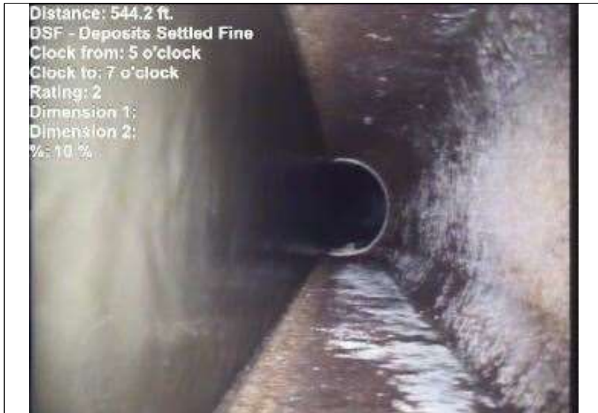
At: 544.2 ft. 5/7 DSF - Deposits Settled Fine Joint: No 10 %
