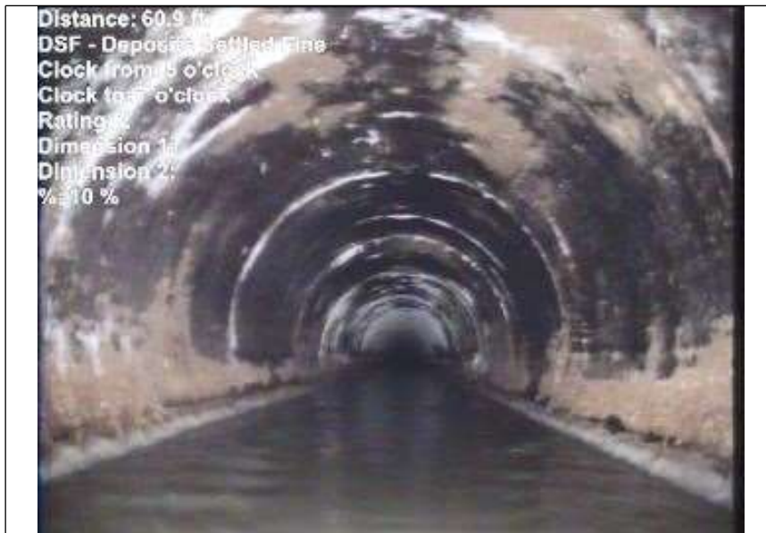
At: 60.9 ft. 5/7 DSF - Deposits Settled Fine Joint: No 10 %
