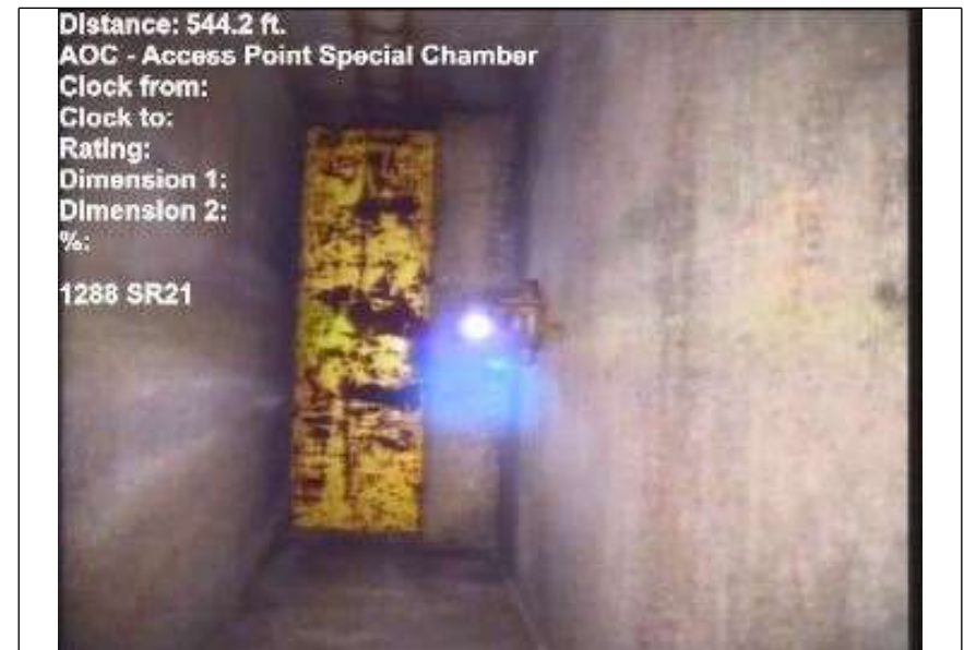
At: 544.2 ft. AOC - Access Point Special Chamber Joint: No 1288 SR21
