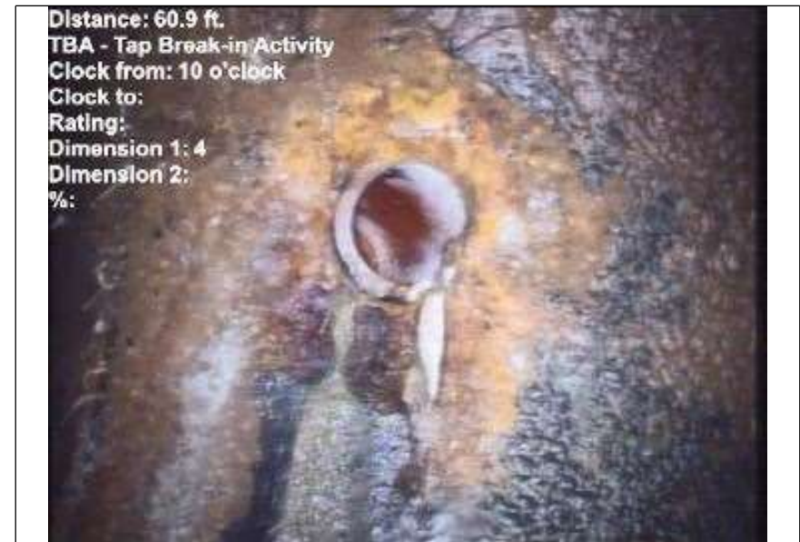
At: 60.9 ft. 10/ TBA - Tap Break-in Activity Joint: No
