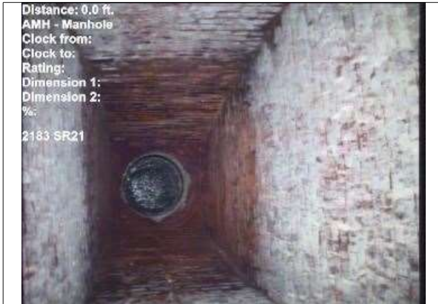
At: 0 ft. AMH - Manhole Joint: No 2183 SR21
