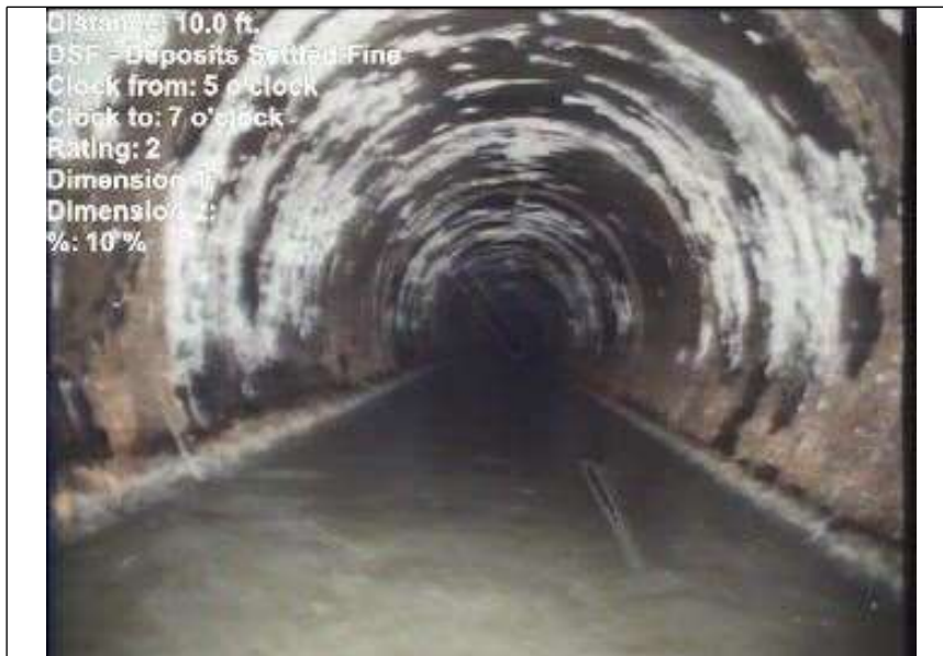
At: 10 ft. 5/7 DSF - Deposits Settled Fine Joint: No 10 %
