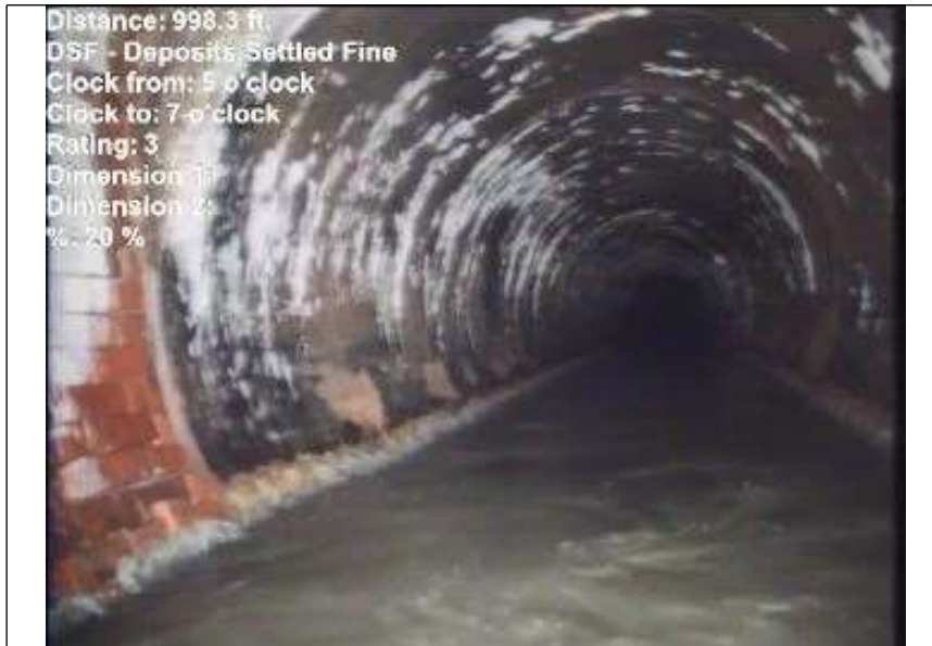
At: 998.3 ft. 5/7 DSF - Deposits Settled Fine Joint: No 20 %
