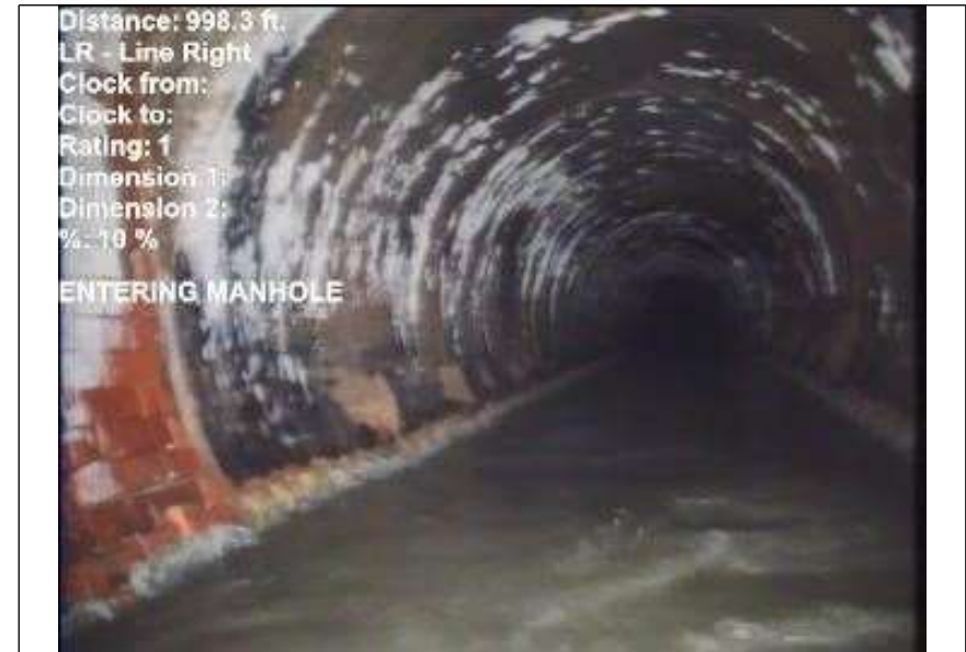
At: 998.3 ft. LR - Line Right Joint: No 10 % ENTERING MANHOLE
