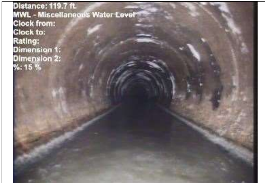
At: 119.7 ft. MWL - Miscellaneous Water Level Joint: No 15 %
