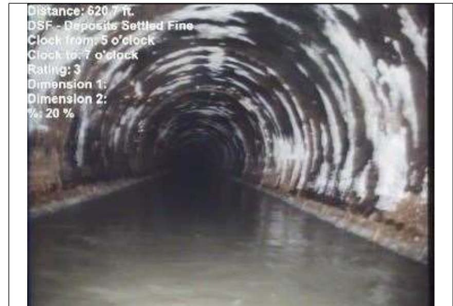
At: 620.7 ft. 5/7 DSF - Deposits Settled Fine Joint: No 20 %
