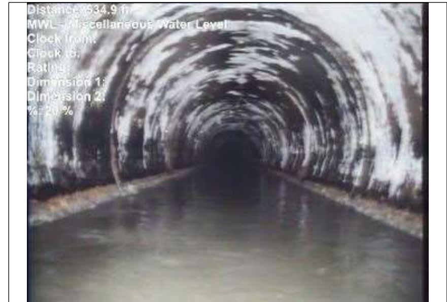
At: 534.9 ft. MWL - Miscellaneous Water Level Joint: No 20 %
