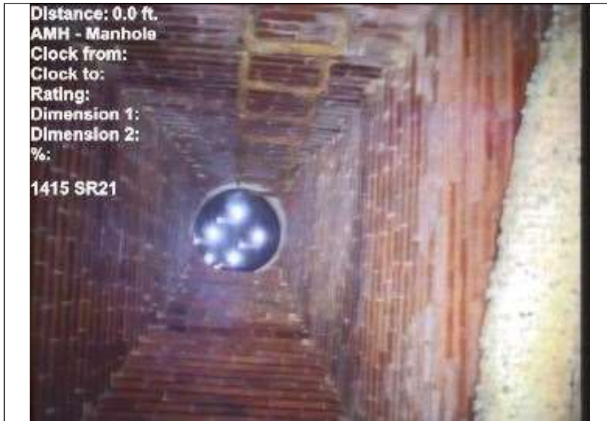
At: 0 ft. AMH - Manhole Joint: No 1415 SR21
