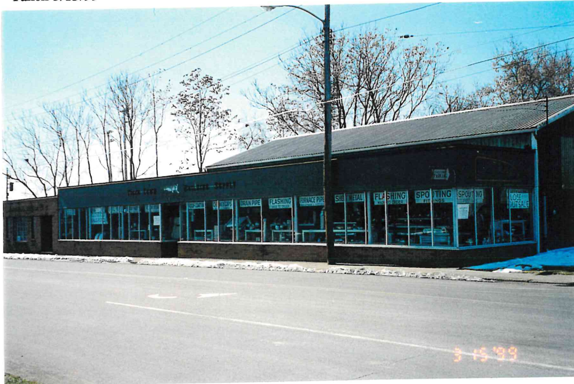
Photograph 1 - View of the front of the property facing northeast.
