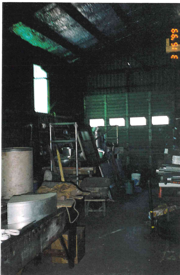
Photograph 6- View of the interior of the garage attached to the building and supply company.
