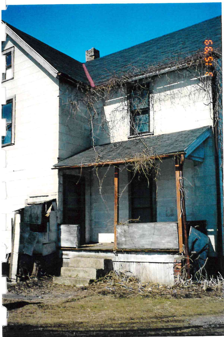
Photograph 5- View of the residence from the Northwest.
