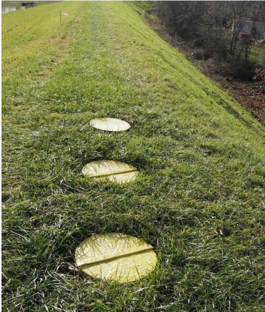
Siphon Breakerss on Levee, James Avenue Pump Station
