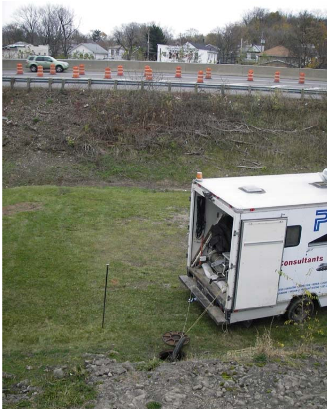
Arch Avenue Storm manhole upstream of levee
