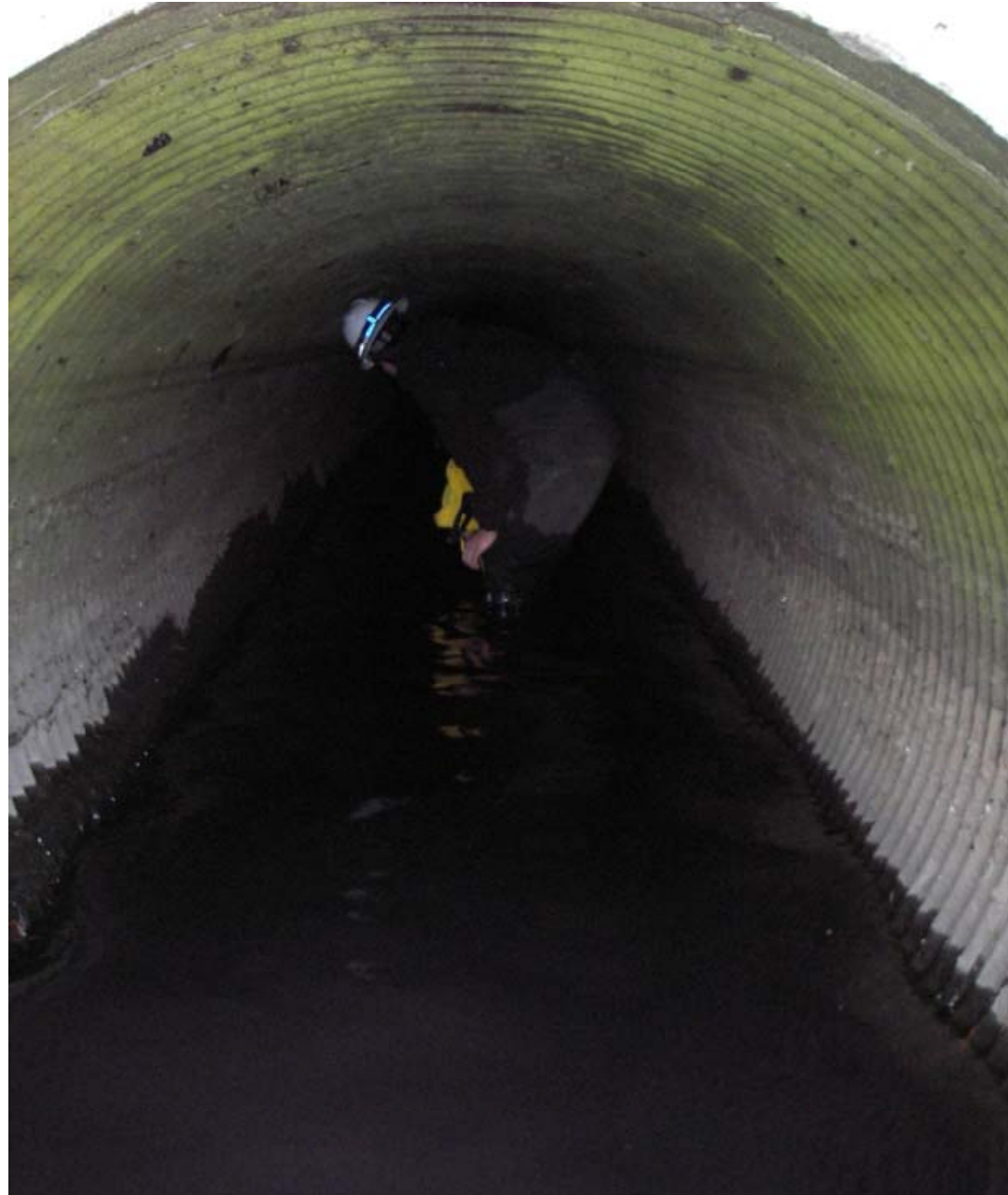
View of entrance at Federal Avenue south pipe
