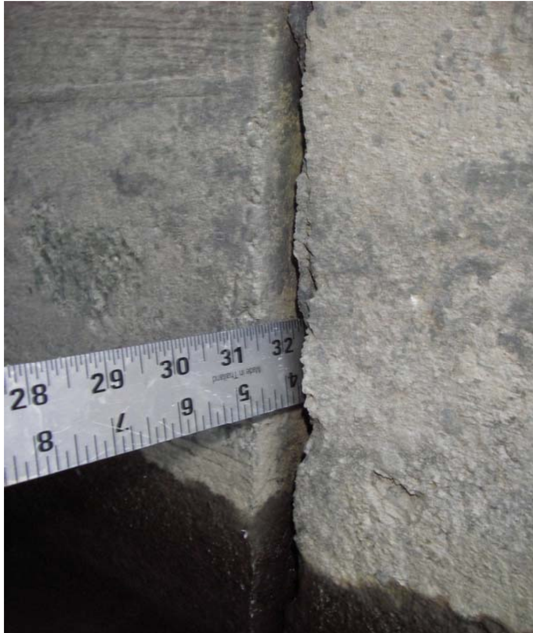
4- inch penetration in right side of box- outlet of box
