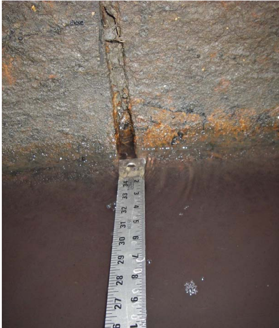
Joint separated, 1-inch, staining at 8:00- 127ft
