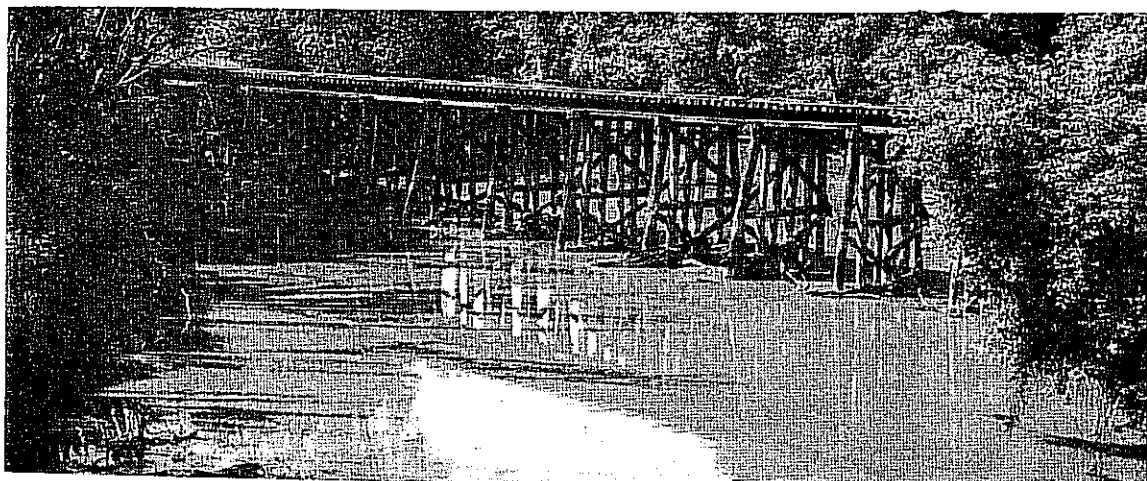
Upstream side of the N.Y.C. & St. L. railroad bridge at Mile 82.15 in Navarre.
