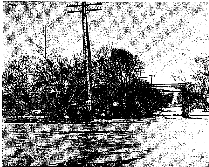
Cherry Road bridge over the Tuscarawas River. This bridge was rebuilt, channel relocated and widened and levees built as a part of the local protection works. Note the buildup of debris on the upstream side of the bridge.
