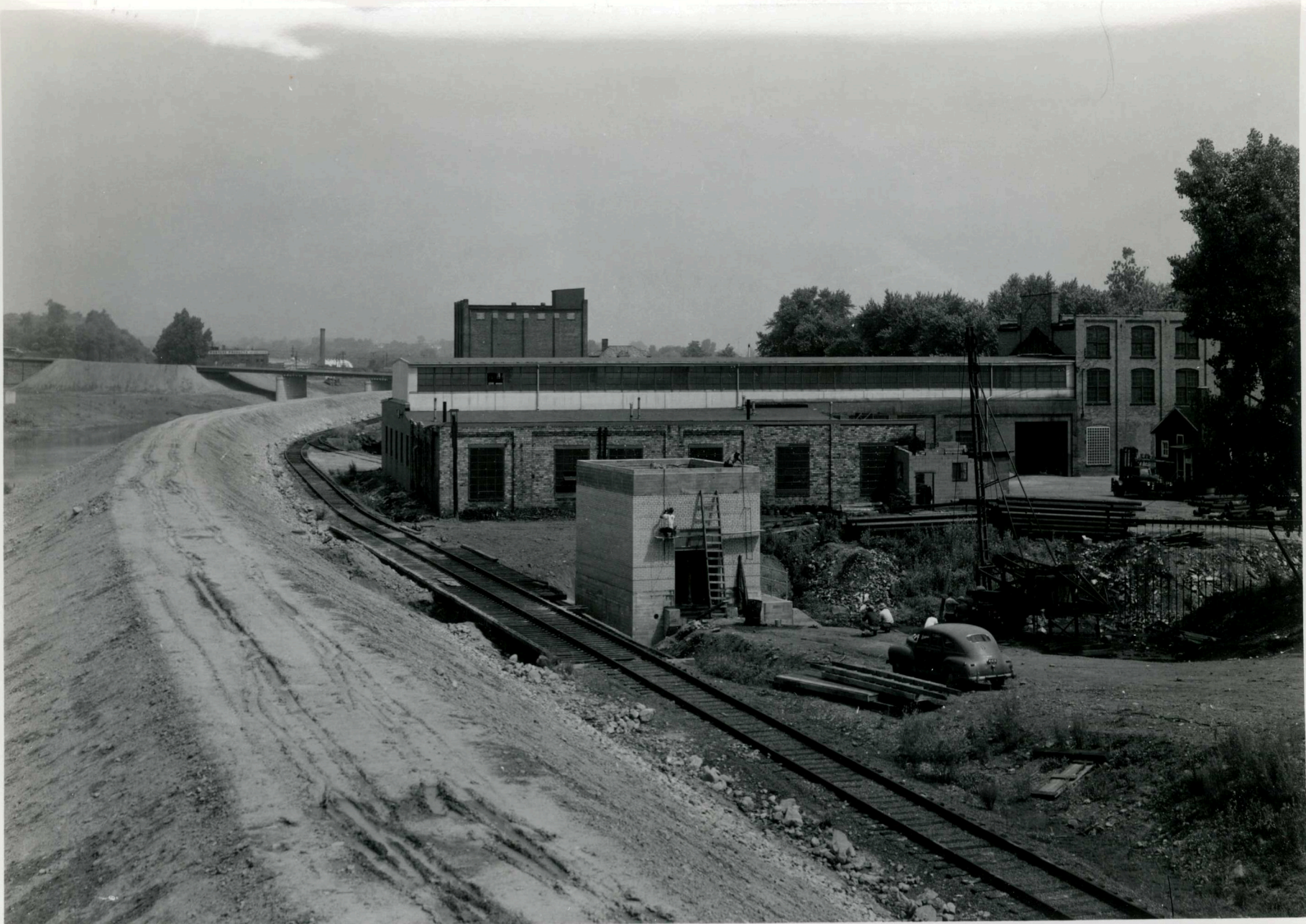
On Lincoln Way at centerline of levee looking upstream showing Federal Avenue Pump Station after completion of motor floor.
