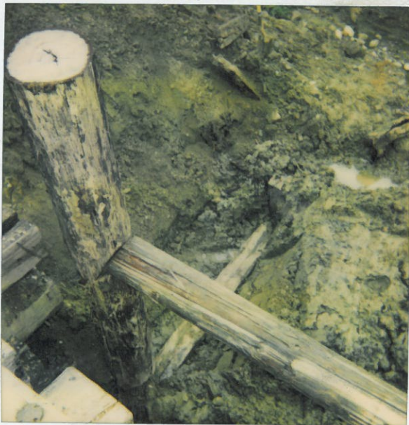
N.W. Corner Bridge beams
