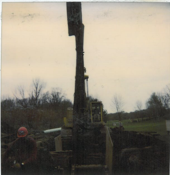
S.W. Corner - East Side Extracted pilings
