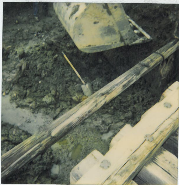
N.E. Corner rail Road tie driving into ground for braising
