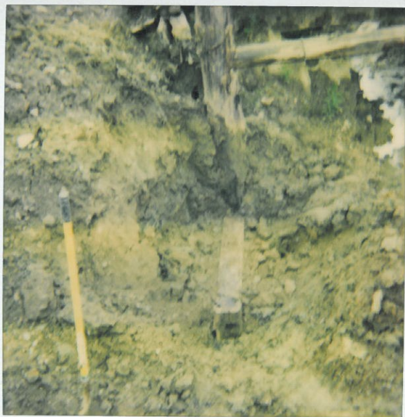
N.E. Corner Bridge Braising
