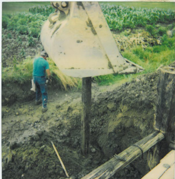
N.E. Driving S.P. Rail Road Tie into ground Corner Bridge Braising
