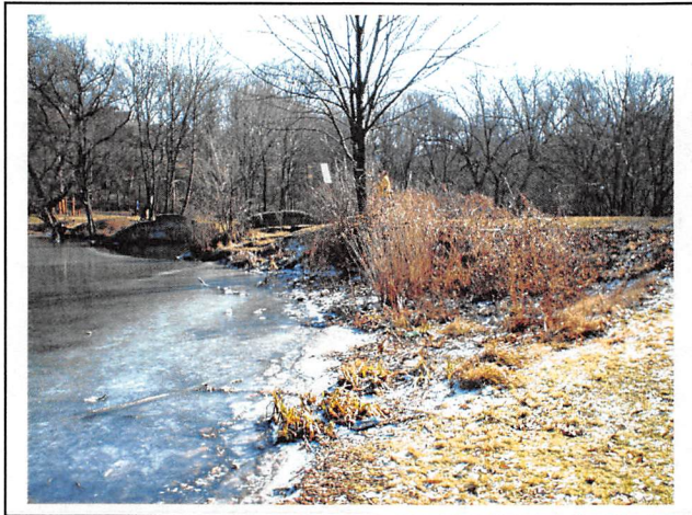
Overview of the upstream slope. Note the trees and brush.
