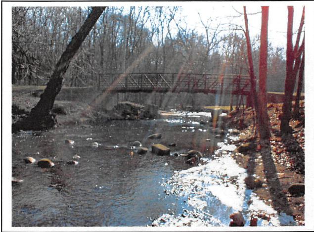
View of the principal spillway outlet channel.
