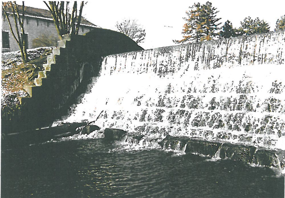
Photo 3 Close-up of spillway showing “steps” which dissipates energy
