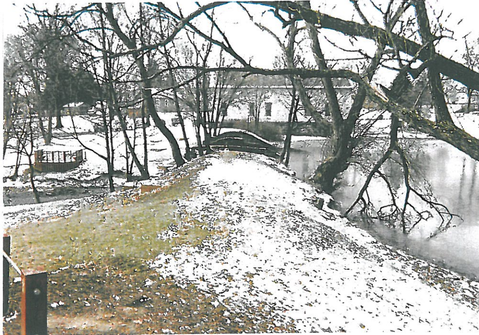
Photo 4 Crest of Earthen Embankment - Looking West
