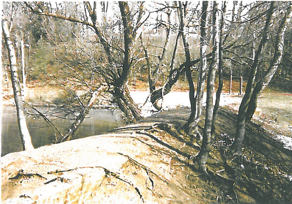
Photo 5 Eastern embankment, note trees and presence of brick wall
