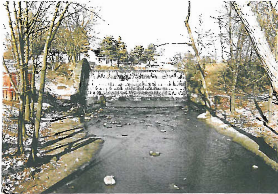
Photo 2 Downstream of Existing Spillway (Rock Weir - 36' in Width)
