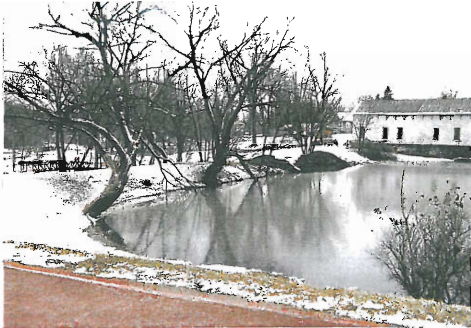
Photo 1 Existing Earthen Embankment and Spillway for Sippo Reservoir
