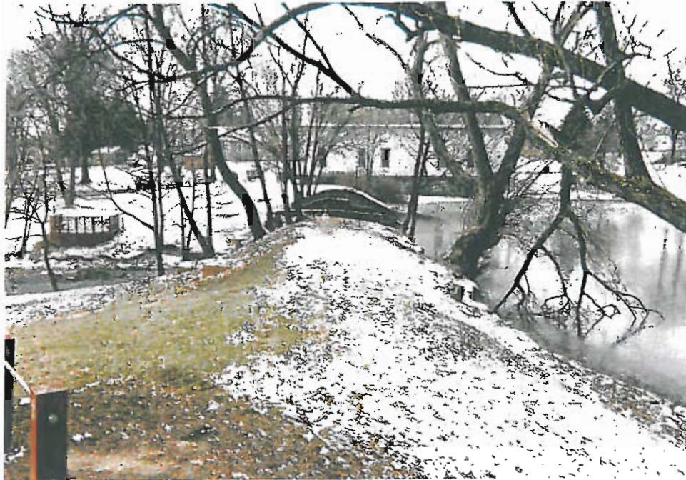
Photo 4 Crest of Earthen Embankment - Looking West
