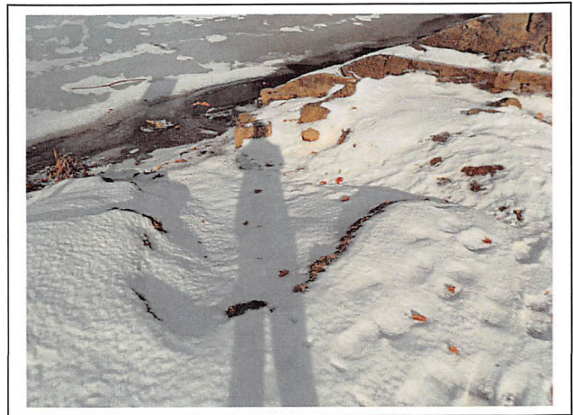
View of the upstream slope that abuts the right principal spillway sidewall in 2016. Though difficult to see because of the snow cover, erosion of the slope has increased.
