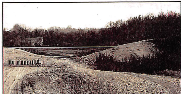
Photograph of dam breach from downstream. White line shows former dam crest.
