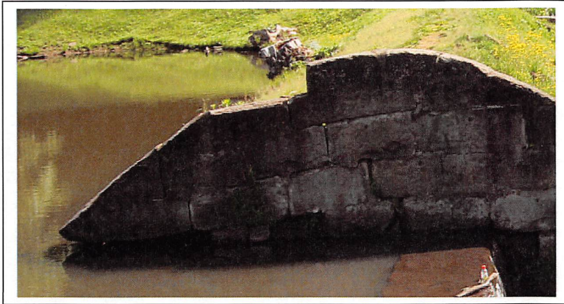
View of left principal spillway side wall in June 2010.
