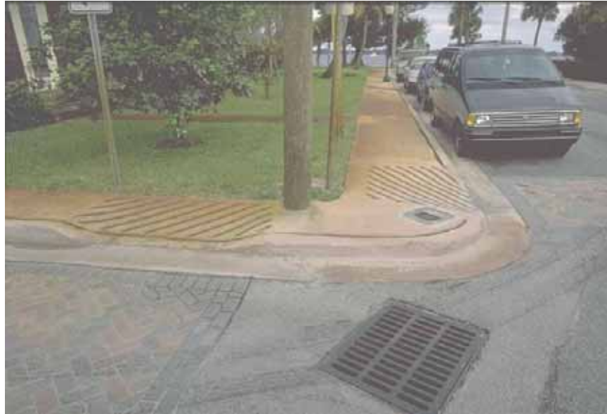
Figure 20-10. Photo. A reduced radius allows for a slower, safer turn.
