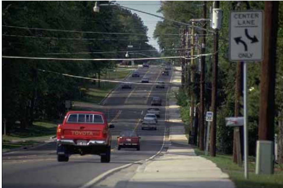
Figure 7-3. Photo. Sidewalks with a landscape strip should be installed to minimize exposure to vehicular traffic.
