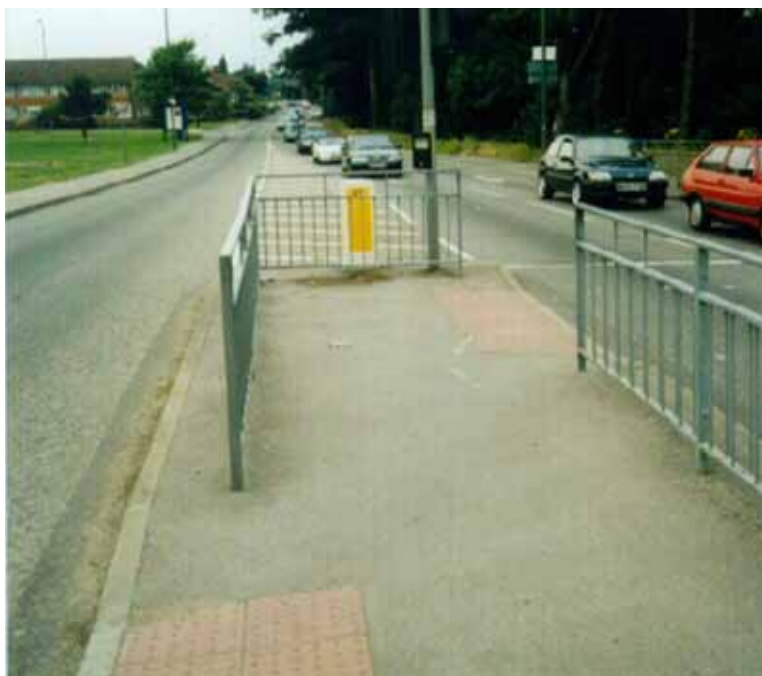
Figure 12-8. Photo. Staggered crosswalk with fencing.
