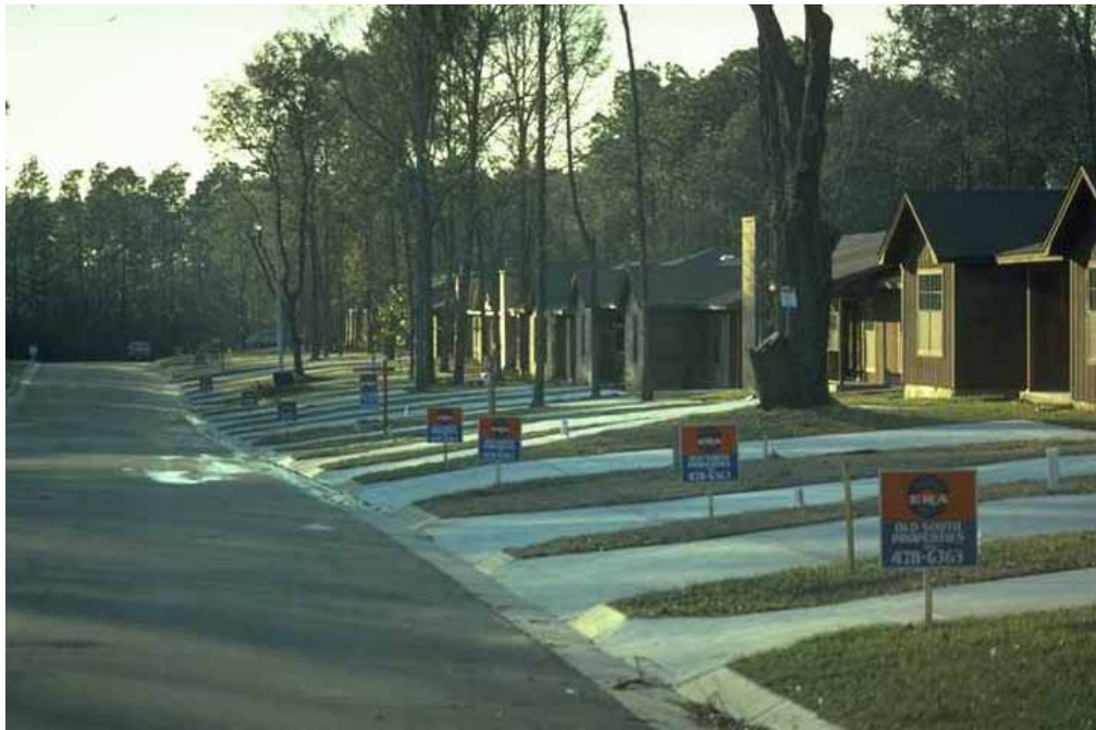
Figure 7-4. Unless required by local ordinance, many developments focus on vehicle access without regard to pedestrian access.
