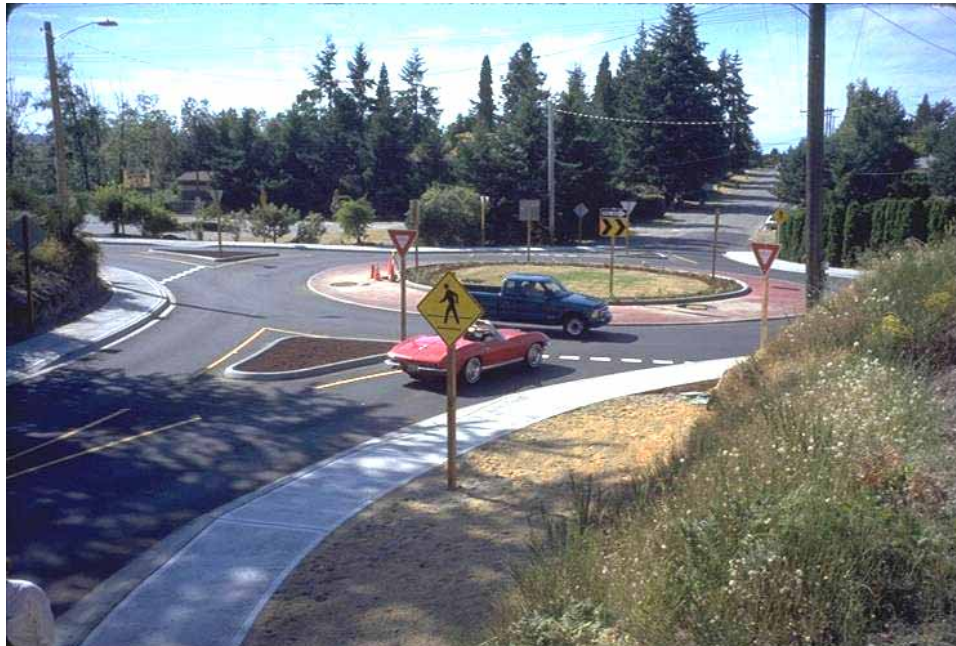
Figure 20-16. Photo. The splitter islands should be raised and landscaped to prevent left-turning vehicles from taking a shortcut across the island.
