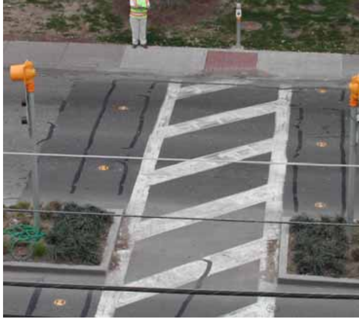
Figure 10-11. Photo. Working example of in-roadway warning lights with pedestrian pushbutton in Austin, Texas.
