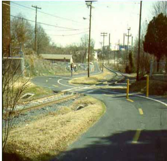
Figure 19-2. Photo. Shared-use paths can be adjacent to railroad lines (Libba Cotton Trail, Carrboro, NC).
