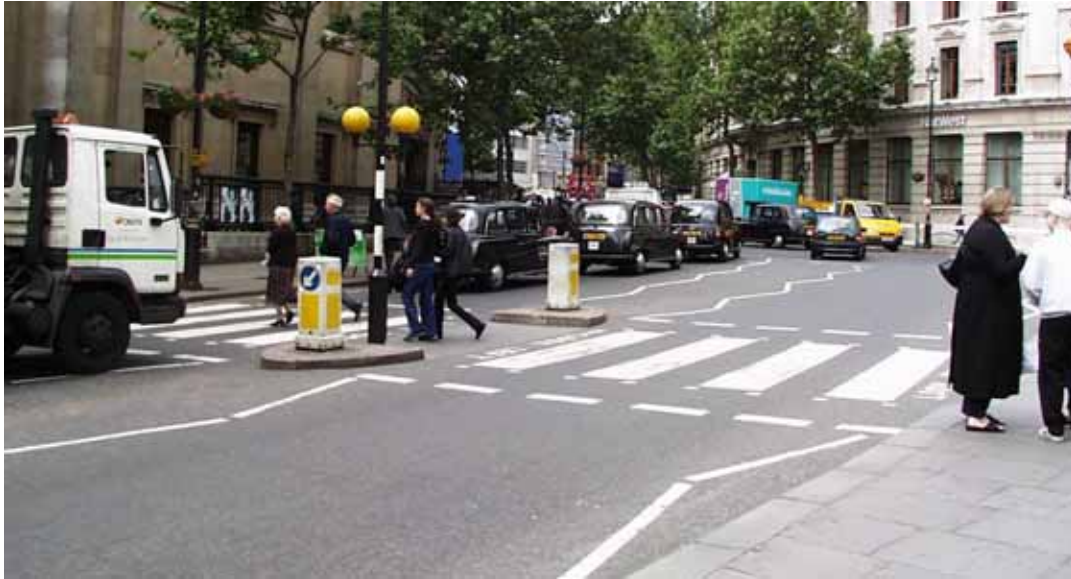
Figure 23-2. Photo. Zebra crossing in London, U.K., with zigzag approach markings and Belisha beacons.
