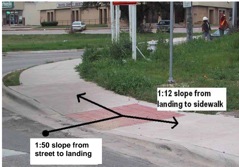
Figure 8-16. Photo. Parallel curb ramp.
