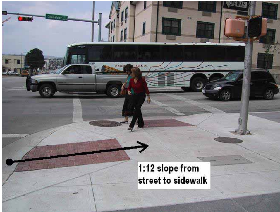
Figure 8-15. Photo. Perpendicular curb ramp.
