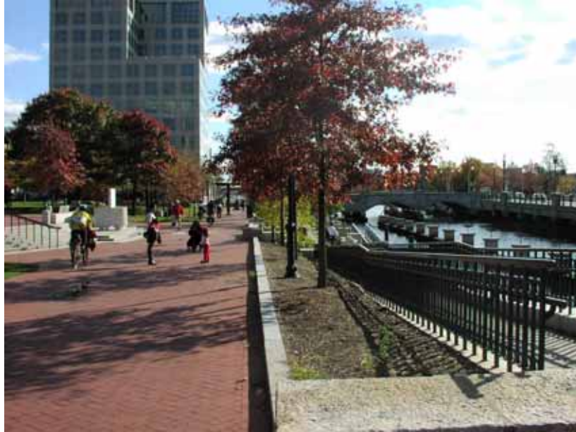
Figure 19-3. Photo. Shared-use paths can be integrated into urban waterfronts and parks, providing direct access to central business districts (East Bay Bicycle Path, Providence, RI).
