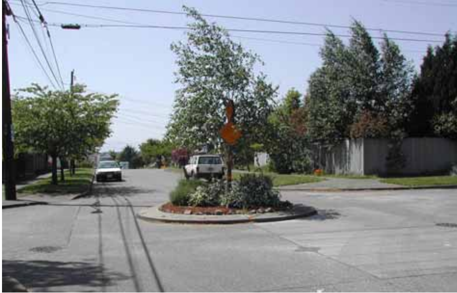
Figure 20-15. Photo. Traffic circles can be designed to accommodate large vehicles and emergency access without undue restrictions.
