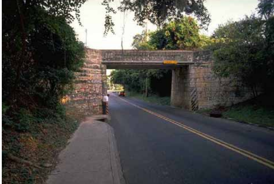
Figure 22-4. Photo. Example of a sidewalk ending at a bridge abutment with no warning or alternative path.
