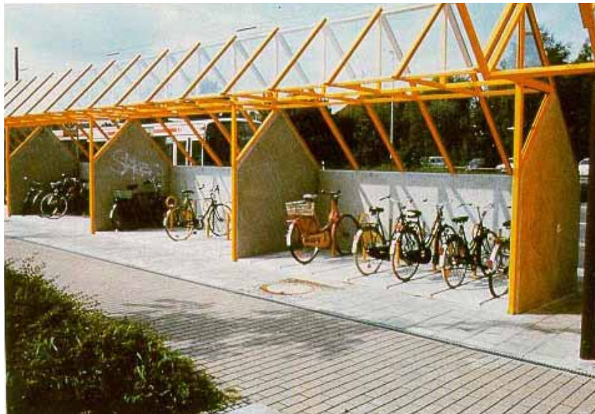
Figure 23-15. Photo. Example of bicycle shelters located at a transit station in Germany.
