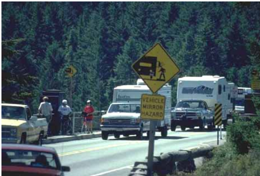
Figure 22-6. Photo. Use of signing to warn motorists and pedestrians of the potential hazard posed by vehicle mirrors on narrow bridge sidewalks.
