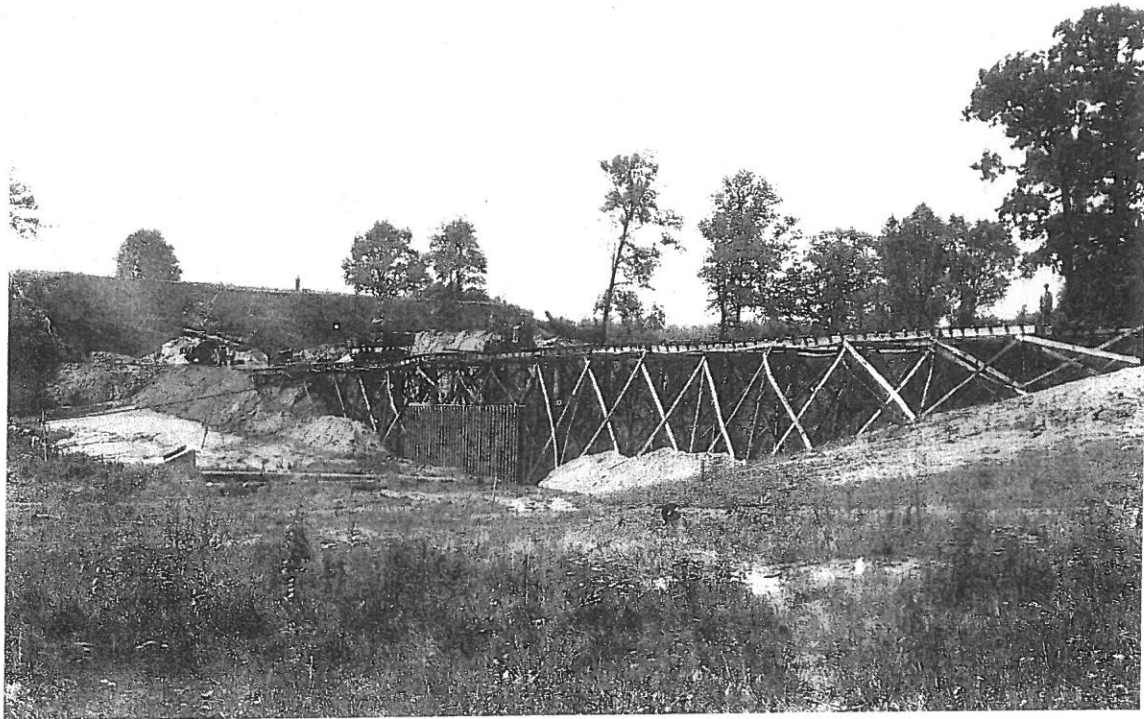
Top: Building the reservoir dam and spillway in 1886, now Sippo Park in Massillon. Massillon Museum Collection
