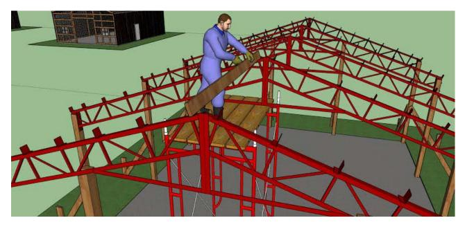
The outermost truss clip will need to be adjusted for a vertical alignment.
