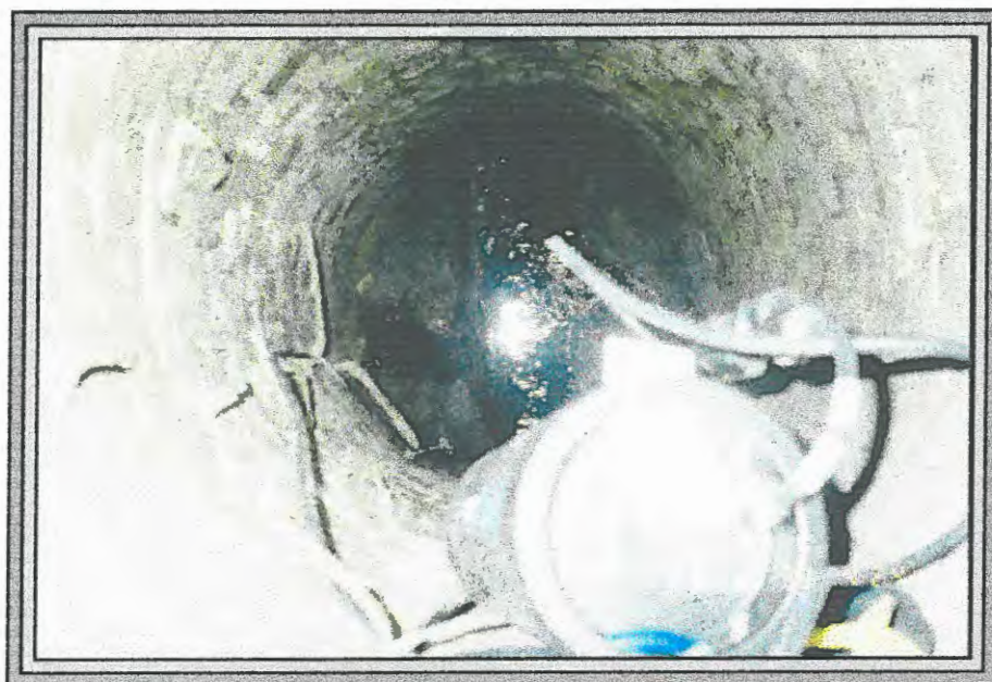
View looking into manhole
