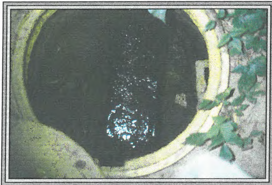
View looking into manhole
