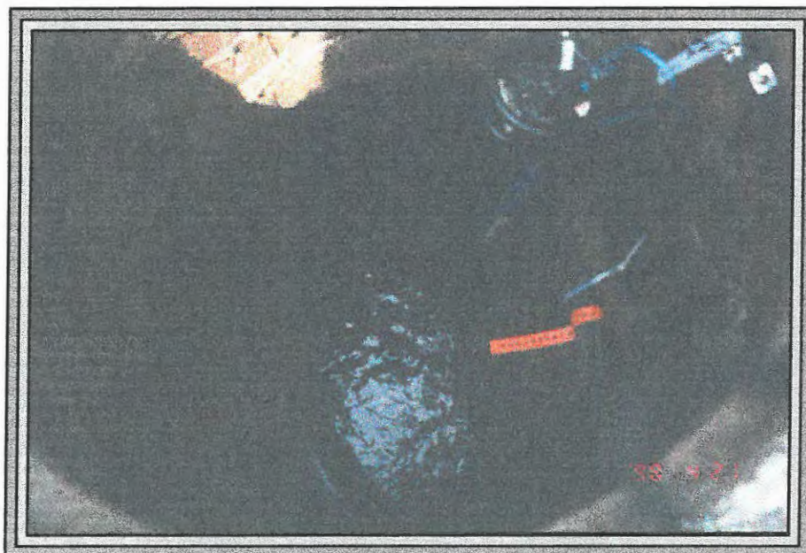
View looking into manhole
